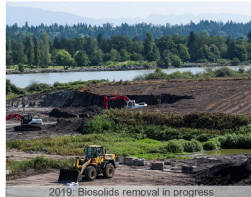
2019: Biosolids removal in progress
