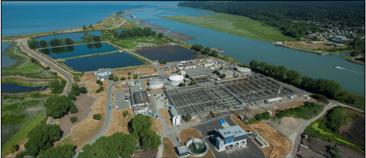
Iona Island Wastewater Treatment Plant
