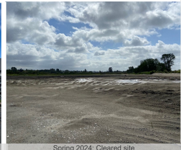
Spring 2024: Cleared site
