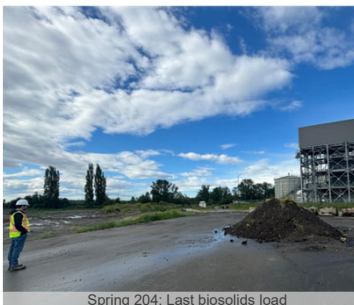
Spring 2024: Last biosolids load
