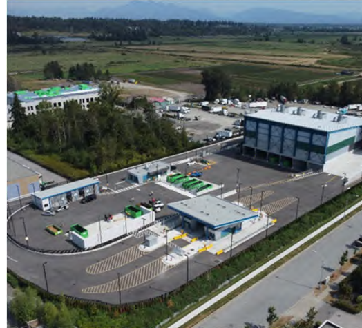
Central Surrey Recycling and Waste Centre
