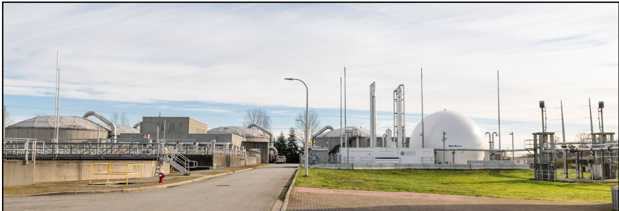
Lulu Island Wastewater Treatment Plant
