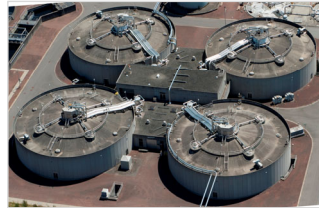
Annacis WWTP Digesters
