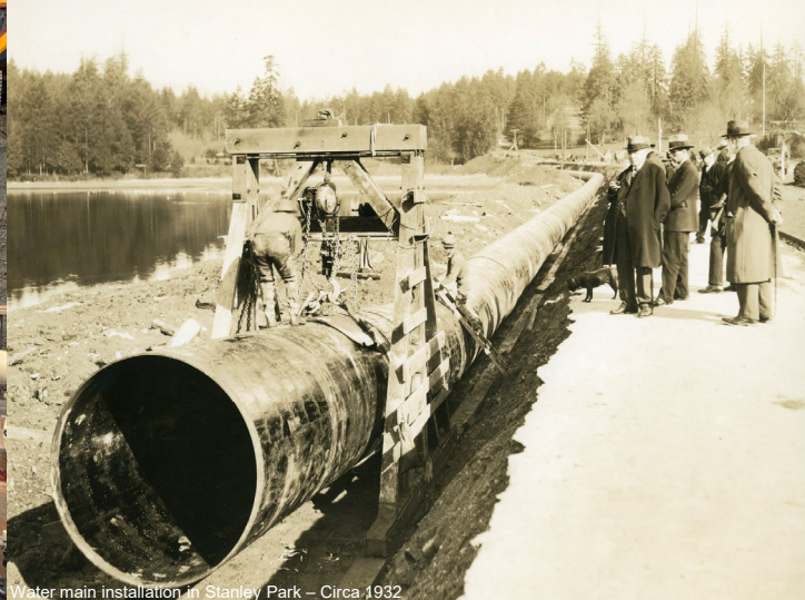
Water main installation in Stanley Park – Circa 1932
