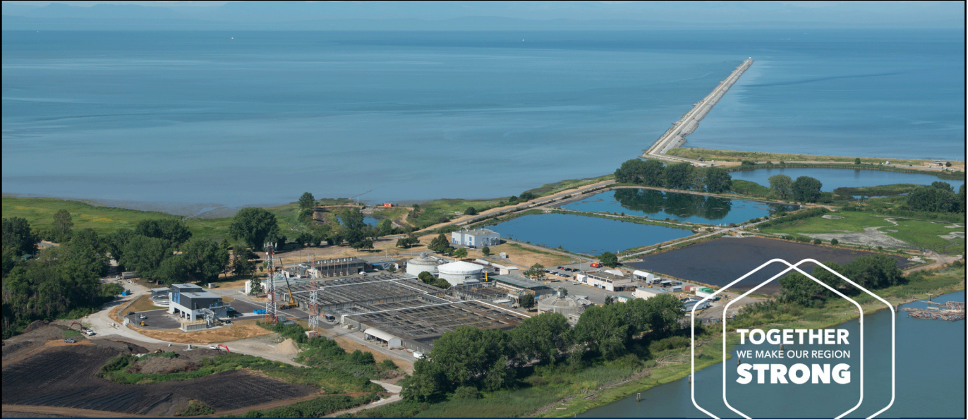
Iona Island Wastewater Treatment Plant
