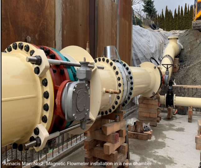
Annacis Main No. 2, Magnetic Flowmeter installation in a new chamber
