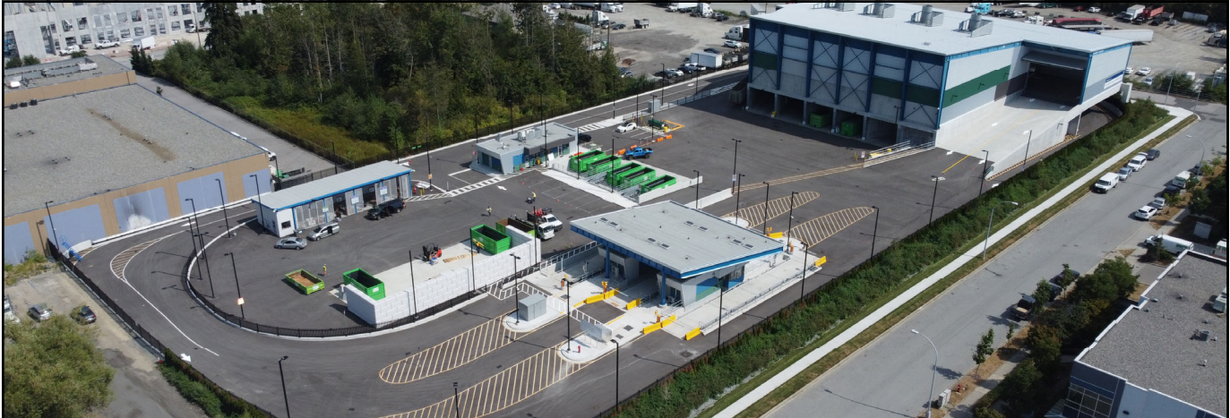
Central Surrey Recycling and Waste Centre
