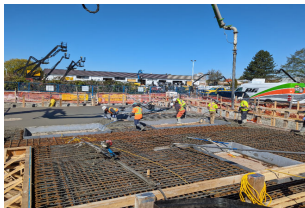
Fleetwood Reservoir Roof slab
