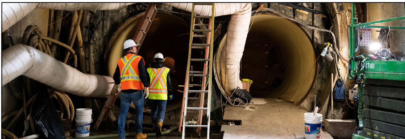
Second Narrows Water Supply Tunnel under construction
