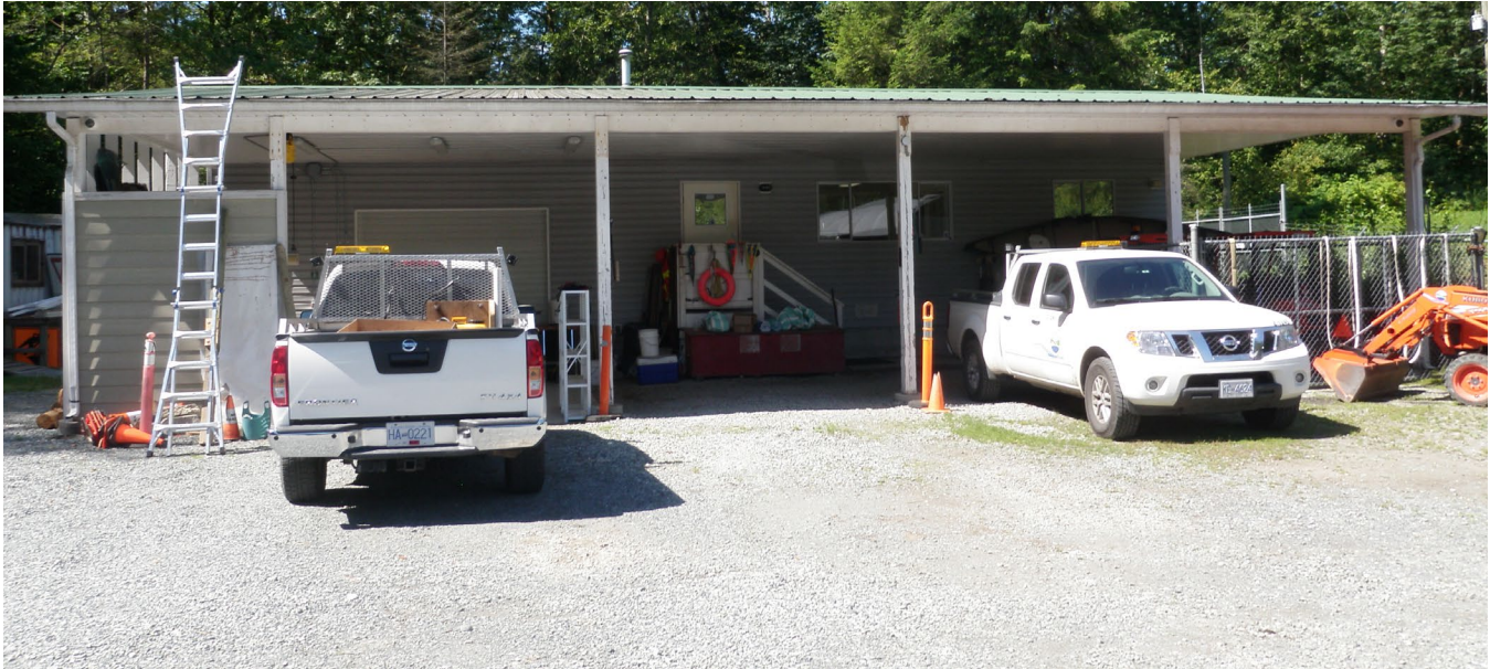
Kanaka Creek Regional Park - Operations Building
