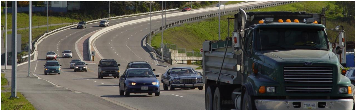
Scott Road transportation corridor, Surrey.
