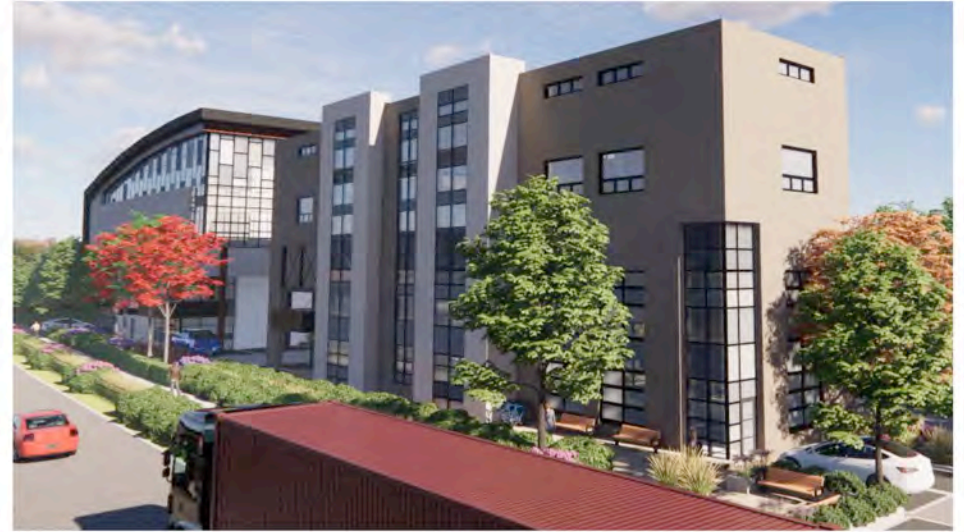
2 VIEW TO SITE FROM 64 AVE LOOKING SOUTH EAST Scale: NTS
