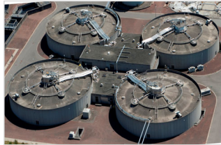
Annacis WWTP Digesters
