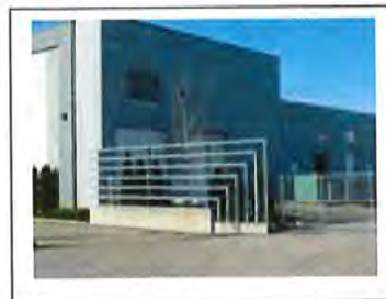
Screening of service and loading areas
