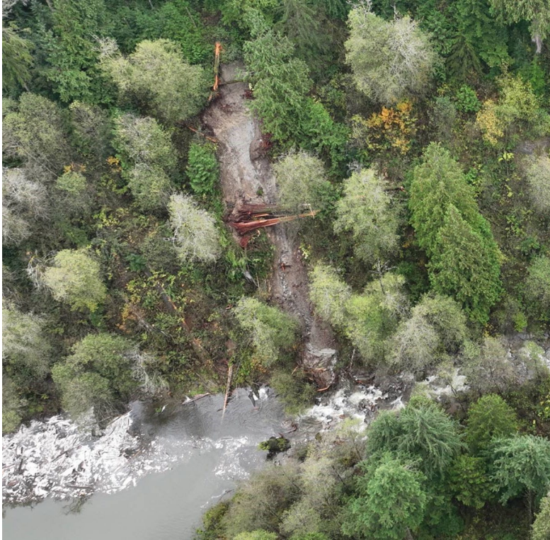
Beaver Creek Washout
