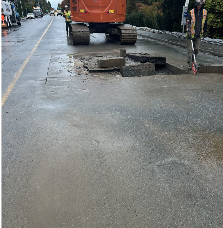
Blundell Sewer, Richmond
