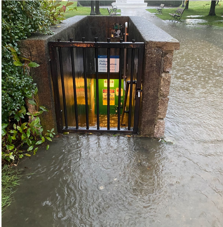
Chilco Pump Station, Stanley Park
