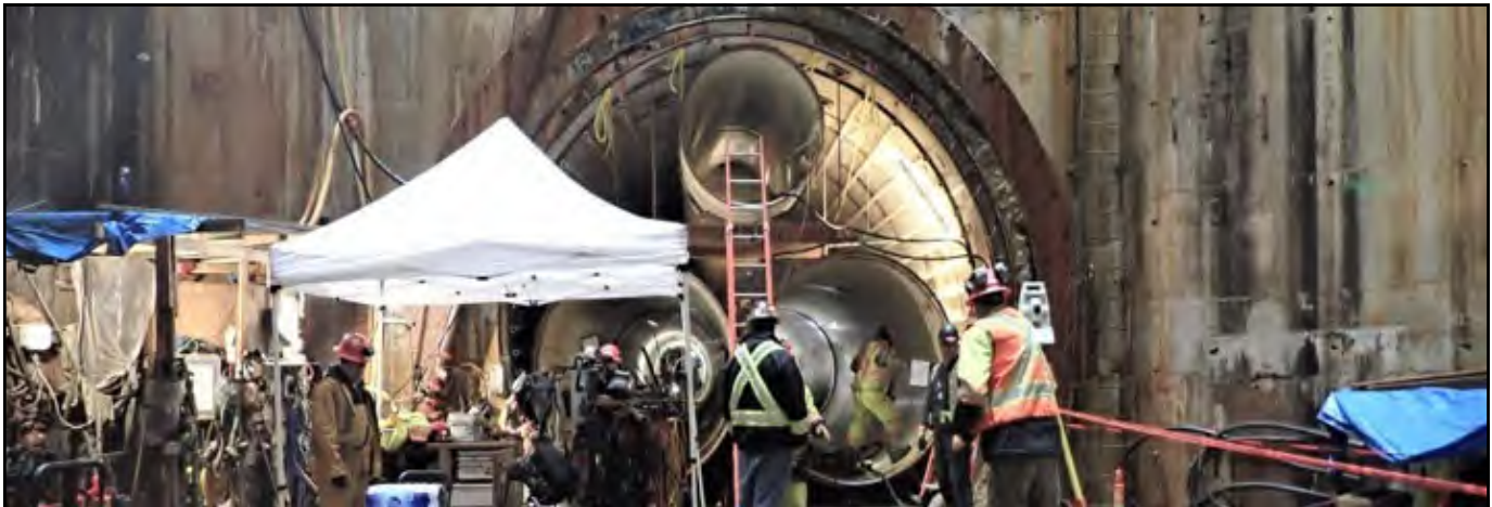
Second Narrows Water Supply Tunnel
