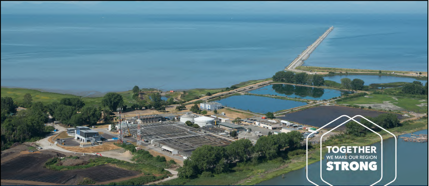
Iona Island Wastewater Treatment Plant
