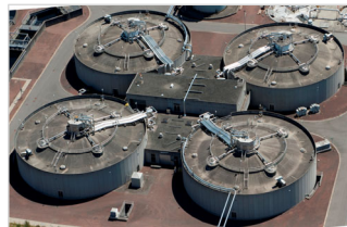
Annacis WWTP Digesters
