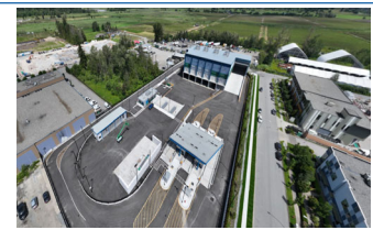
Central Surrey Recycling and Waste Centre
