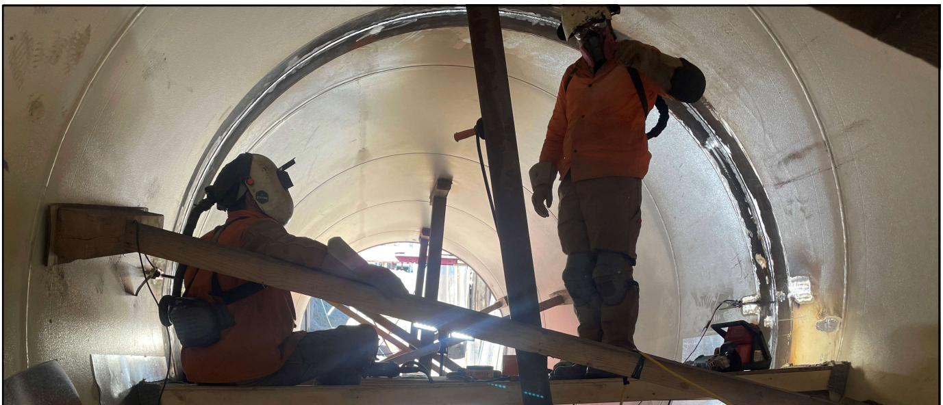
Crew inside the Coquitlam Water Main No. 4 during construction
