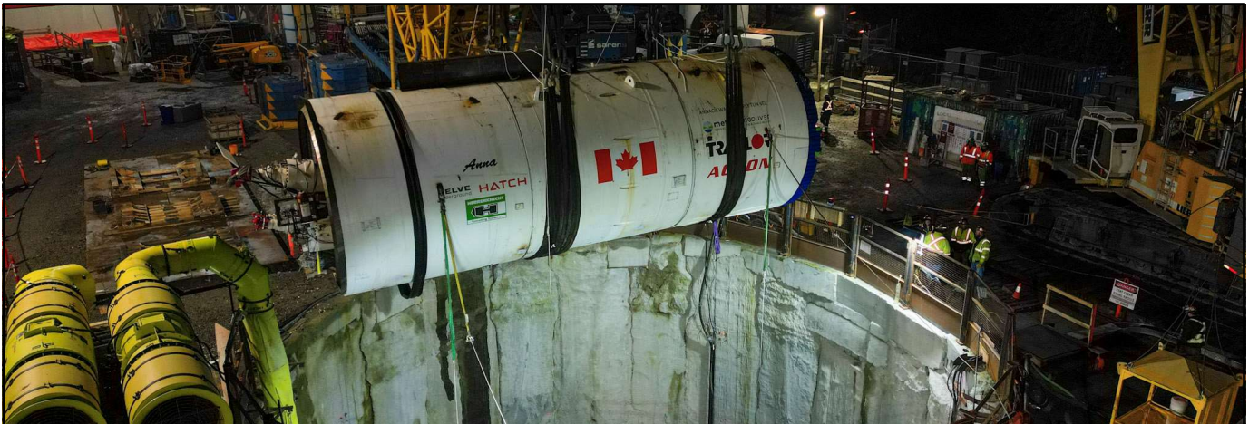
Annacis Water Supply Tunnel
