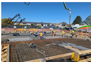
Fleetwood Reservoir roof slab
