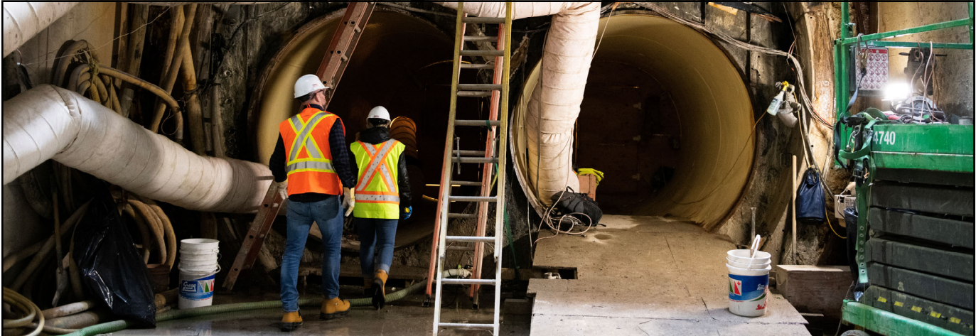
Inside the Second Narrows Water Supply Tunnel during construction
