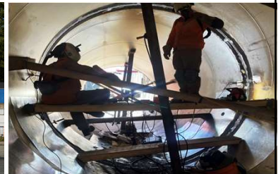
Coquitlam Water Main construction underway
