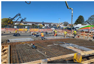
Fleetwood Reservoir Roof slab
