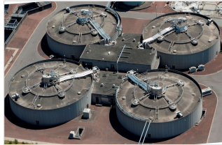
Annacis WWTP Digesters
