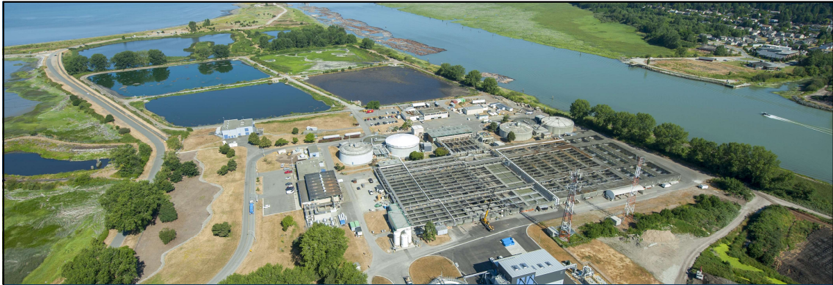
Iona Island Wastewater Treatment Plant
