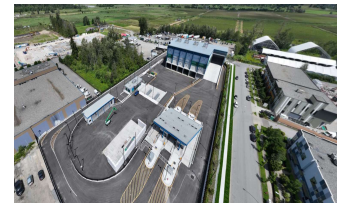
Central Surrey Recycling and Waste Centre
