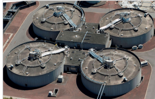
Annacis WWTP Digesters
