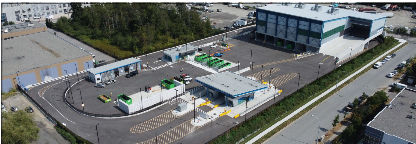
Central Surrey Recycling and Waste Centre
