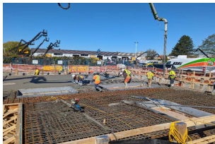
Fleetwood Reservoir roof slab
