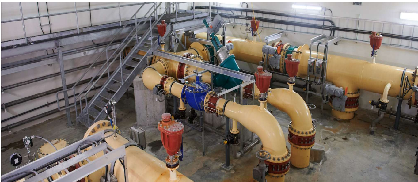
Clayton Reservoir Valve Chamber
