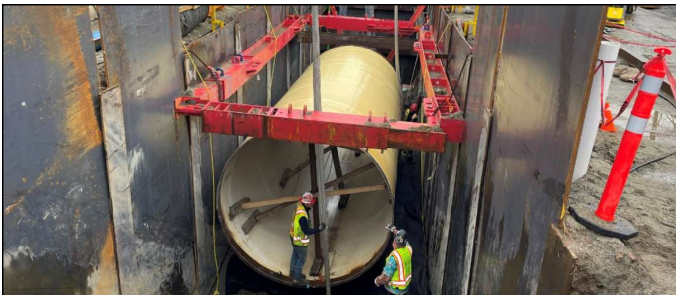
Coquitlam Water Main Construction
