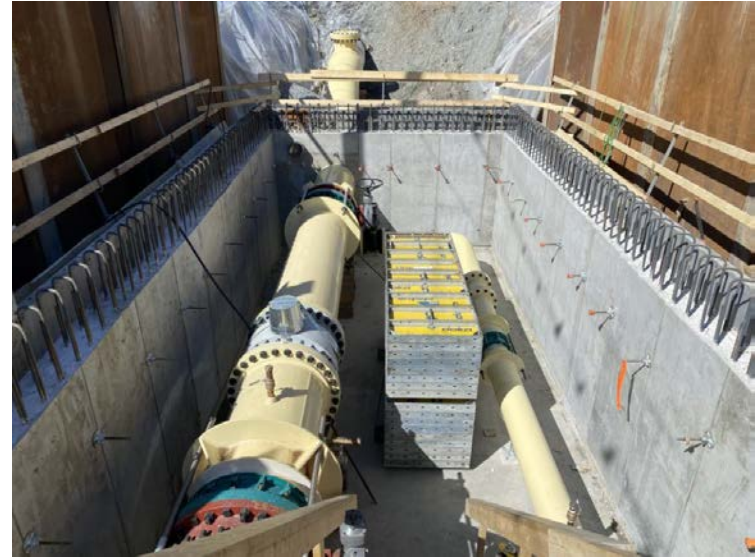
New magnetic meter installation M194 on Annacis Main#2
