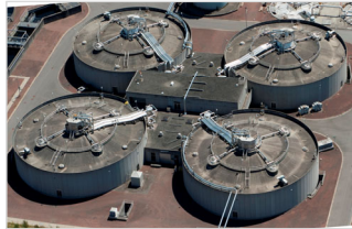
Annacis WWTP Digesters
