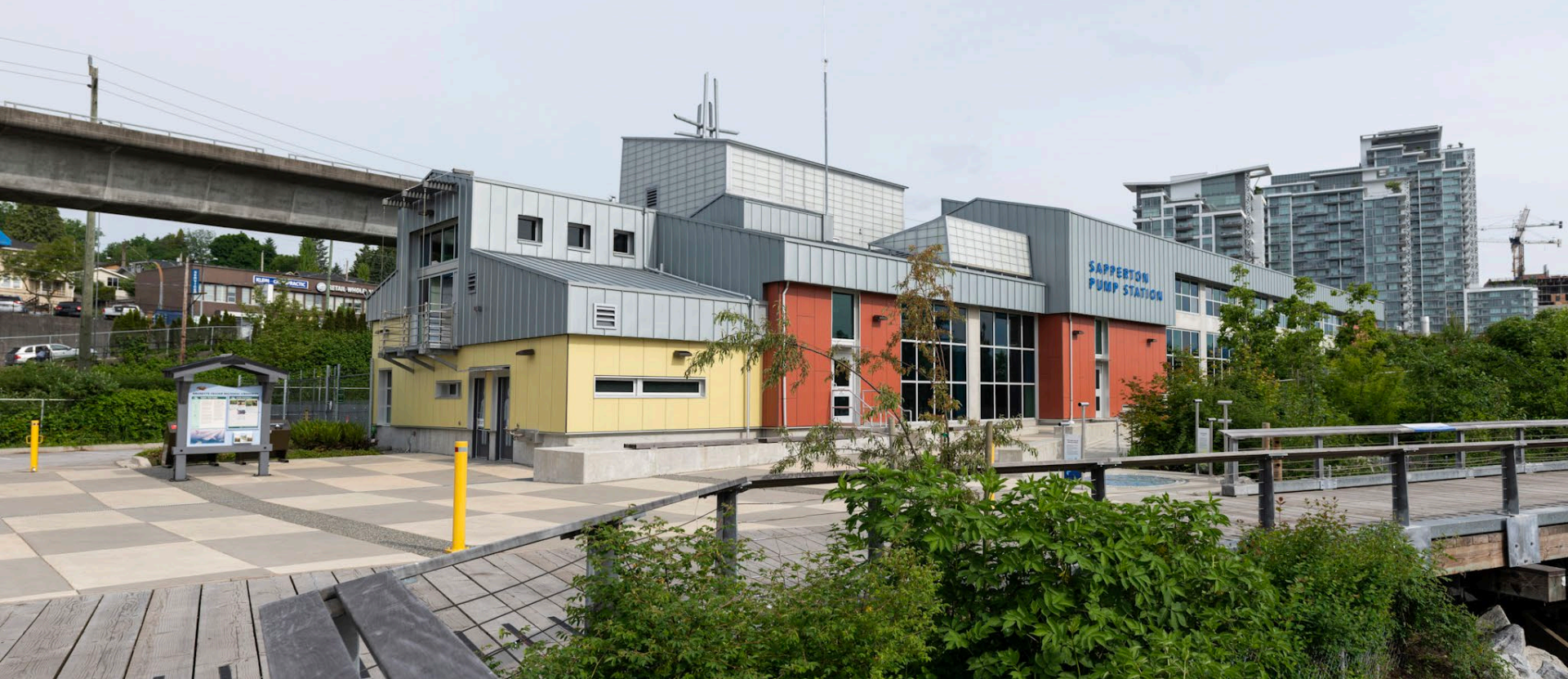
Sapperton Pump Station
