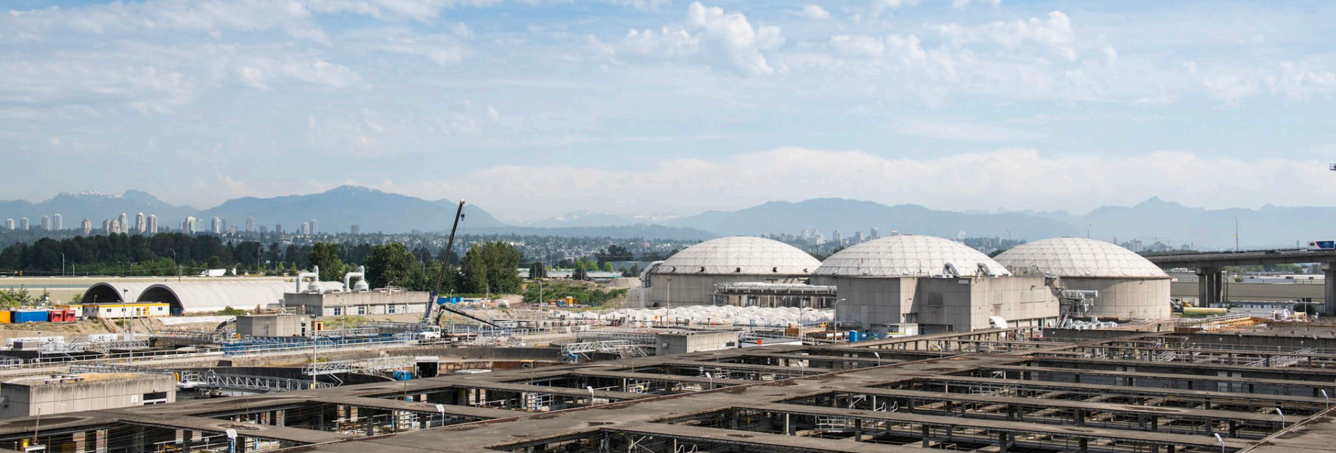
Annacis Island Wastewater Treatment Plant
