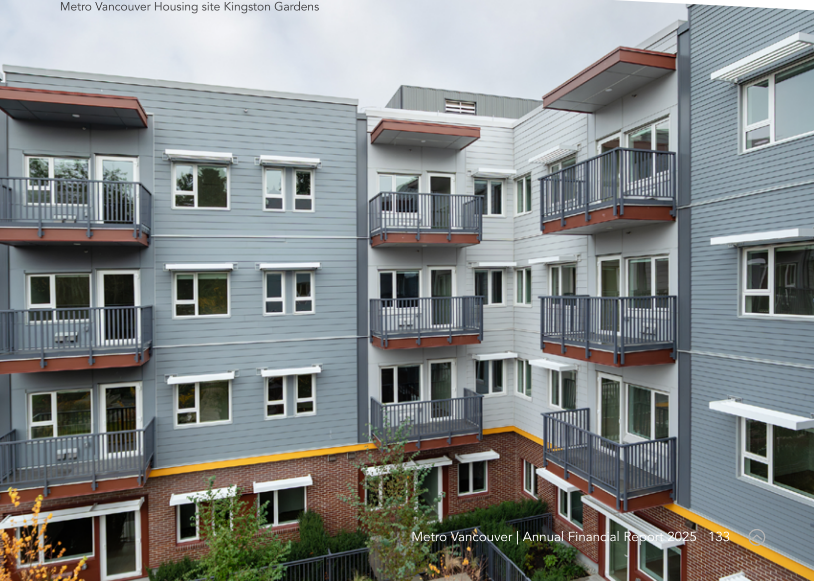
Metro Vancouver Housing site Kingston Gardens
