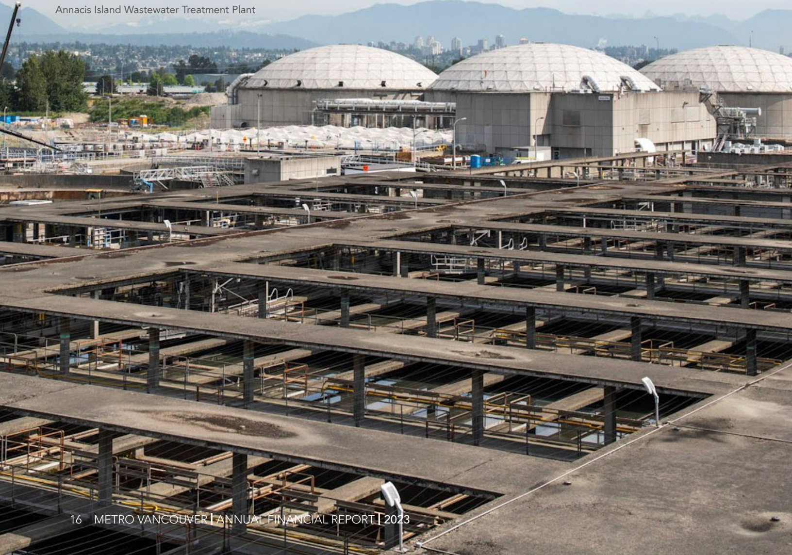
Annacis Island Wastewater Treatment Plant
