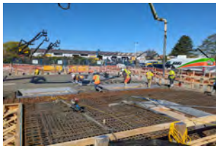
Fleetwood Reservoir Roof slab
