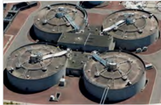
Annacis WWTP Digesters
