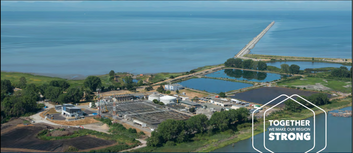
Iona Island Wastewater Treatment Plant
