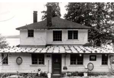
The Bole House in 1950. (Ralph Drew)
