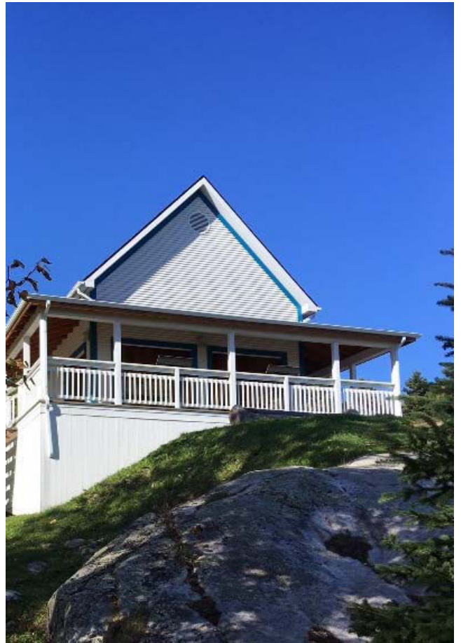
access to porch
